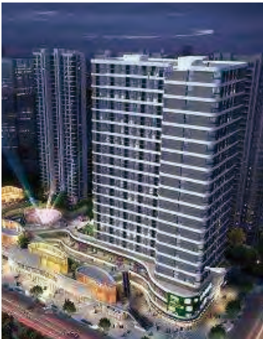
Apartment 金地下沙公寓
