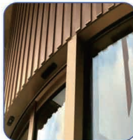
Anti pinch sensor of revolving door
