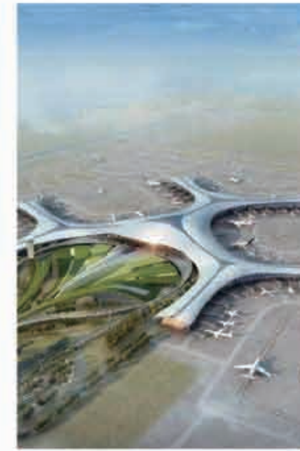
Dalian Shihezi International Airport
